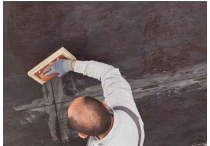
fig.39 / Grouting.
