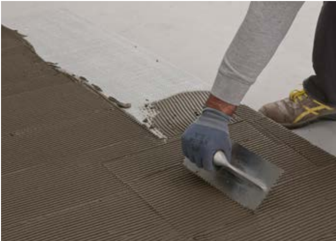
fig.36 / Application of the adhesive on the slab back side.
