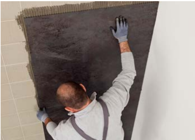
fig.38 / Application of the slab.
