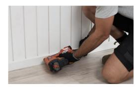
• Lastly, install skirting boards, cornices and dado rails as necessary.
